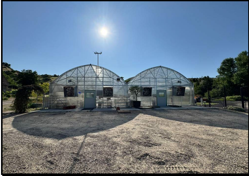
The view of the subject looking east.
